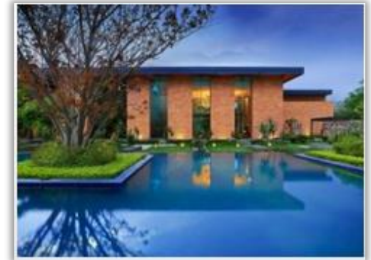
Taj Vivanta, Damdama, Gurgaon
